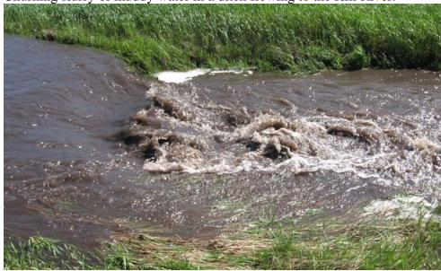
o Massive washout of a tall embankment and its side-water-inlet culvert(s) along the Hill River, east of Brooks along Hwy 92.
